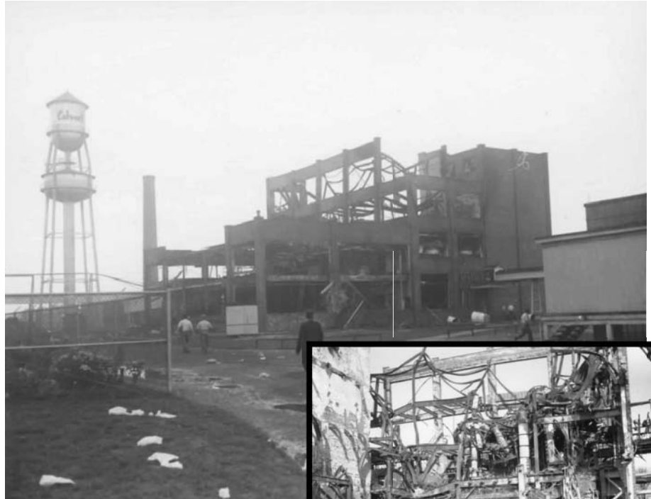
View of the distillery building following the fire.
